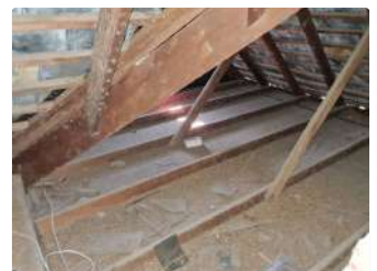
Ref #5 - Roof Structure
