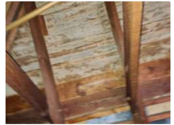
Ref #5 - Roof Structure
