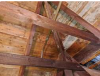
Ref #5 - Roof Structure
