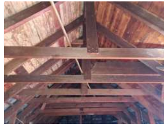
Ref #5 - Roof Structure
