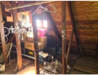
Ref #5 - Roof Structure
