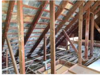
Ref #5 - Roof Structure
