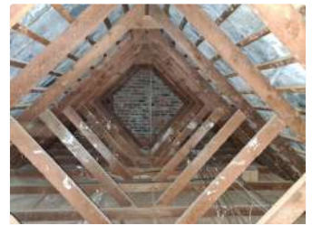
Ref #5 - Roof Structure
