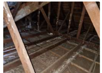
Ref #5 - Roof Structure
