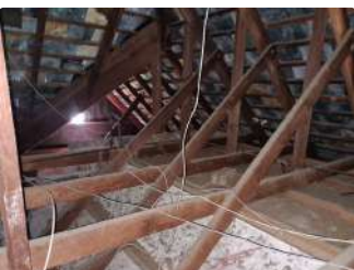
Ref #5 - Roof Structure
