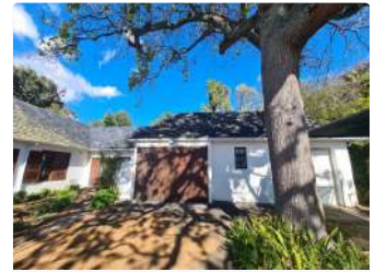
Ref #4 - Roof Covering
