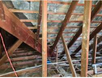
Ref #5 - Roof Structure
