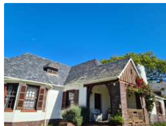
Ref #4 - Roof Covering
