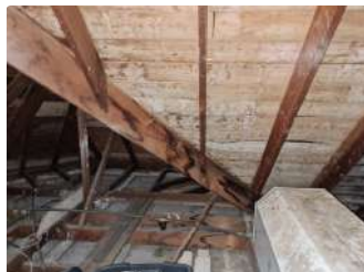
Ref #5 - Roof Structure
