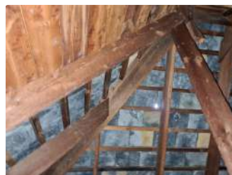
Ref #5 - Roof Structure
