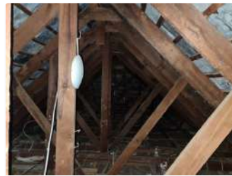
Ref #5 - Roof Structure
