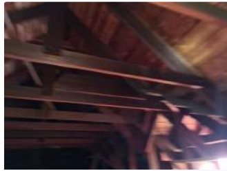
Ref #5 - Roof Structure
