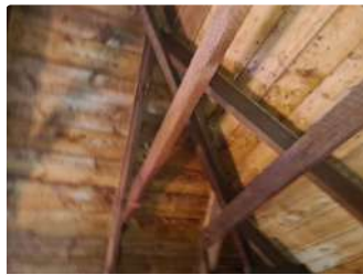
Ref #5 - Roof Structure
