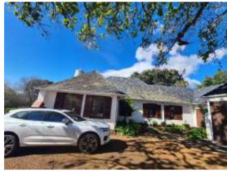
Ref #4 - Roof Covering
