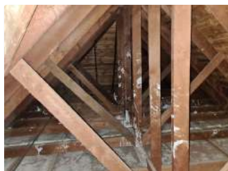
Ref #5 - Roof Structure
