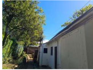
Ref #4 - Roof Covering
