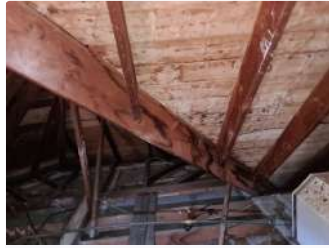
Ref #5 - Roof Structure
