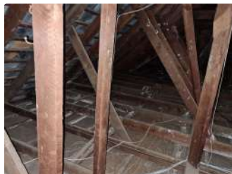
Ref #5 - Roof Structure
