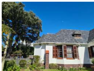
Ref #4 - Roof Covering
