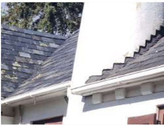
Ref #4 - Roof Covering
