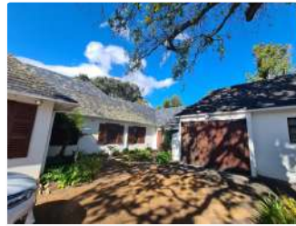
Ref #4 - Roof Covering
