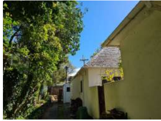
Ref #4 - Roof Covering
