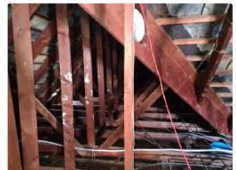
Ref #5 - Roof Structure
