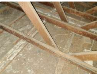
Ref #5 - Roof Structure
