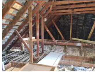
Ref #5 - Roof Structure
