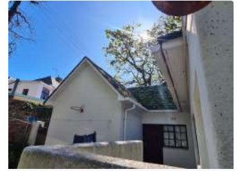
Ref #4 - Roof Covering
