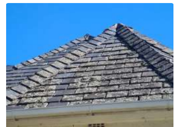
Ref #4 - Roof Covering
