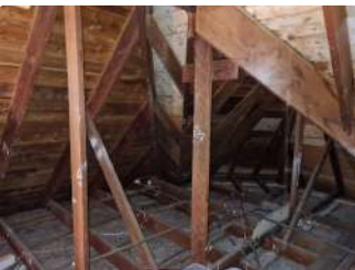
Ref #5 - Roof Structure
