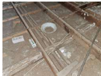
Ref #5 - Roof Structure
