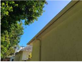
Ref #4 - Roof Covering
