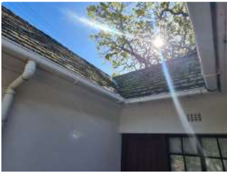
Ref #4 - Roof Covering
