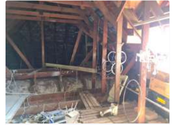
Ref #5 - Roof Structure
