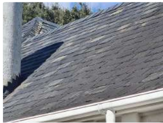
Ref #4 - Roof Covering
