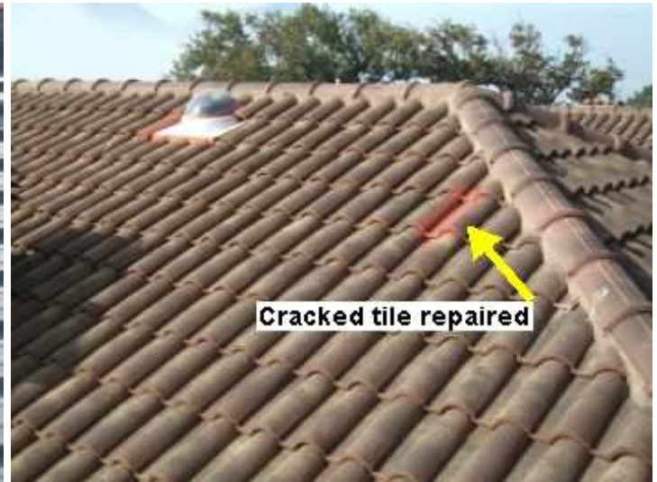
House roof - generally in good condition
