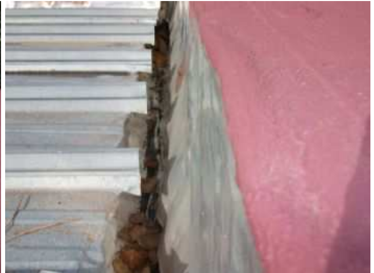
Entrance hall roof - keep gutters clean
