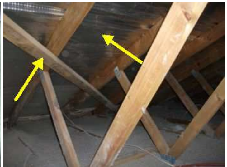
Roof structure - insulation in good condition and bracing correctly installed
