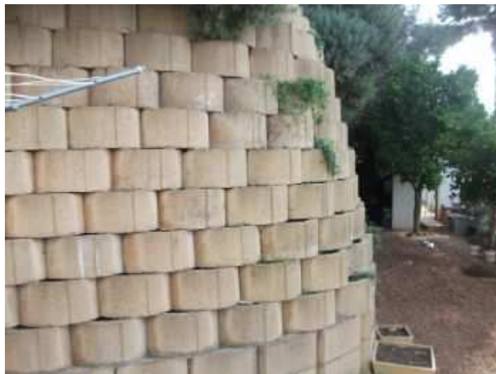
House north side - retaining wall appears to be structurally sound
