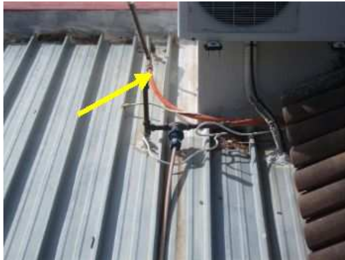
Geyser - hot water supply from geyser should be copper pipe or plastic composite pipe
