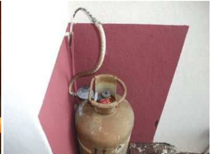
Dining room - external gas installation appears to comply with regulations
