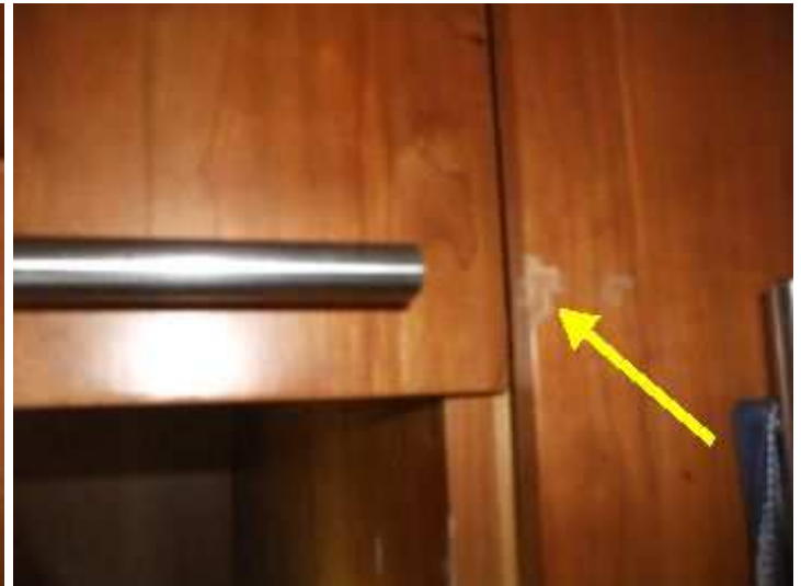
Laundry - general wear and tear marks to some cupboards - doors require realignment
