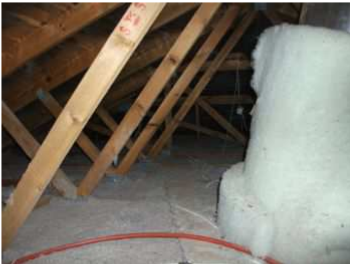
Roof structure - structurally sound and in good condition
