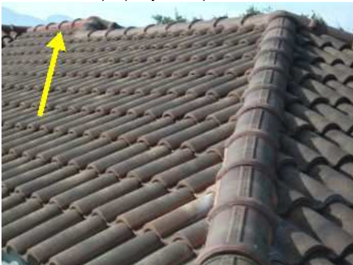
House roof (above main bedroom) - ridges waterproofed
