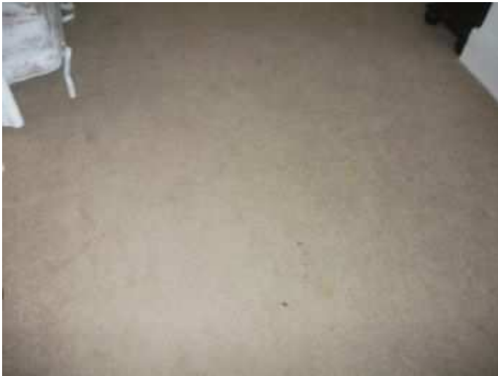
Dining room - carpets with general wear and tear marks
