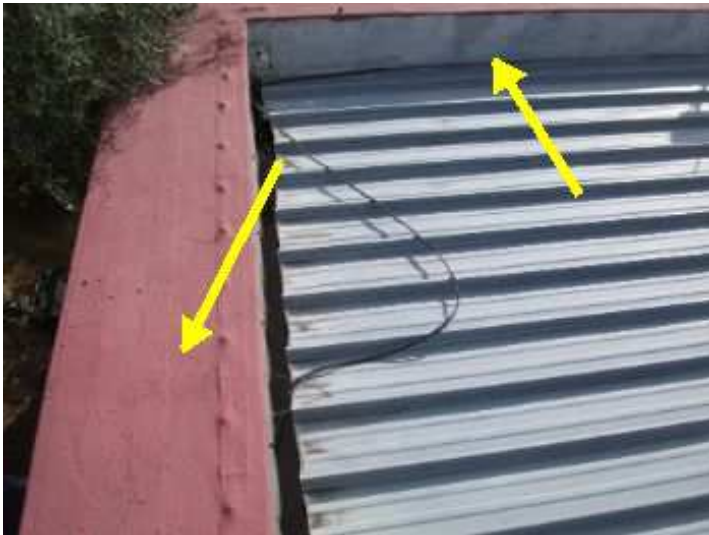
Garage roof - flashings and top of parapet walls properly waterproofed
