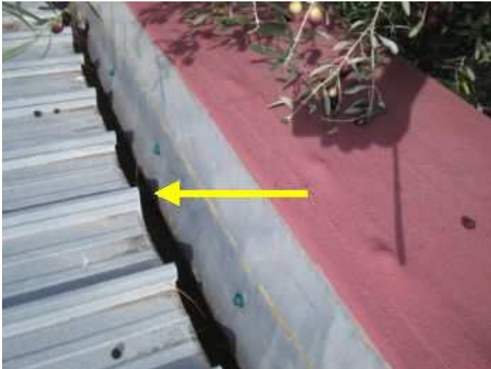
Garage roof - keep gutters clean
