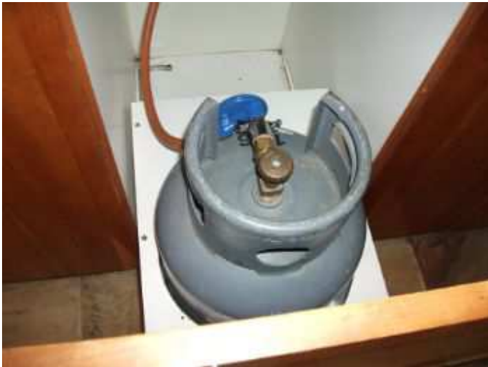
Kitchen - internal gas installation appears to comply with regulations
