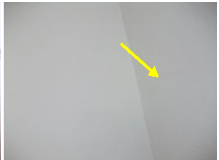
Bedroom 1 north east corner - repaired settlement cracks
